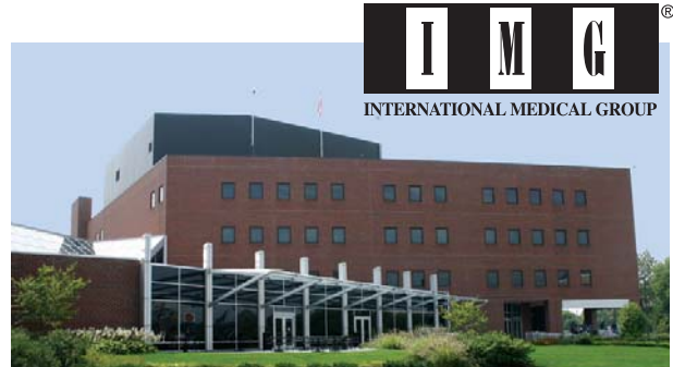
IMG World Headquarters, Indianapolis, Indiana
